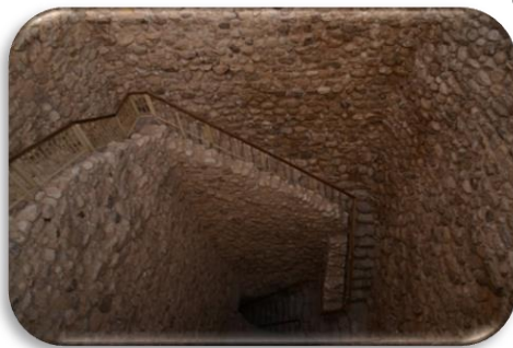
Stairwell down shaft of water reservoir
